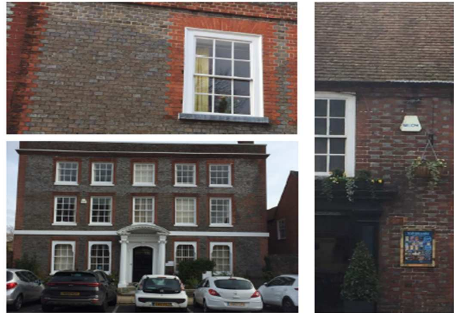
LOCAL BRICKWORK TECHNIQUES
